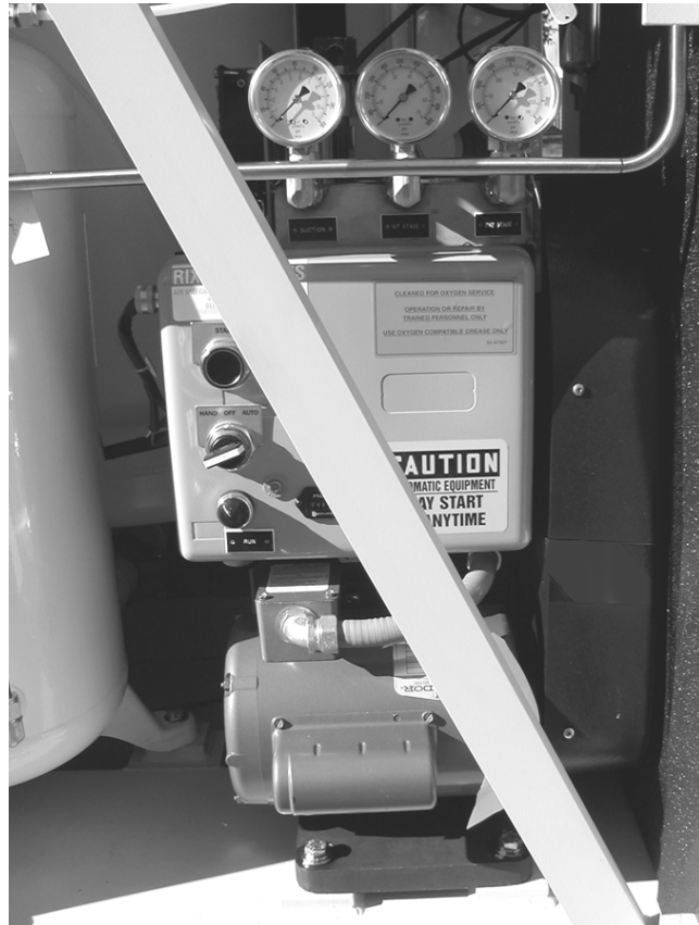
Figure 10. High Pressure Booster Compressor.
