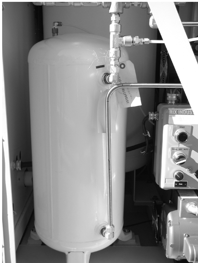
Figure 12. Oxygen Storage Tank (C-500).
