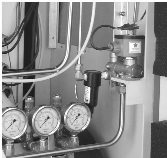
Figure 13. Off-Spec Solenoid Valve (SV-2).
