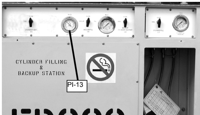
Figure 6. Oxygen Backup Supply System Panel.
