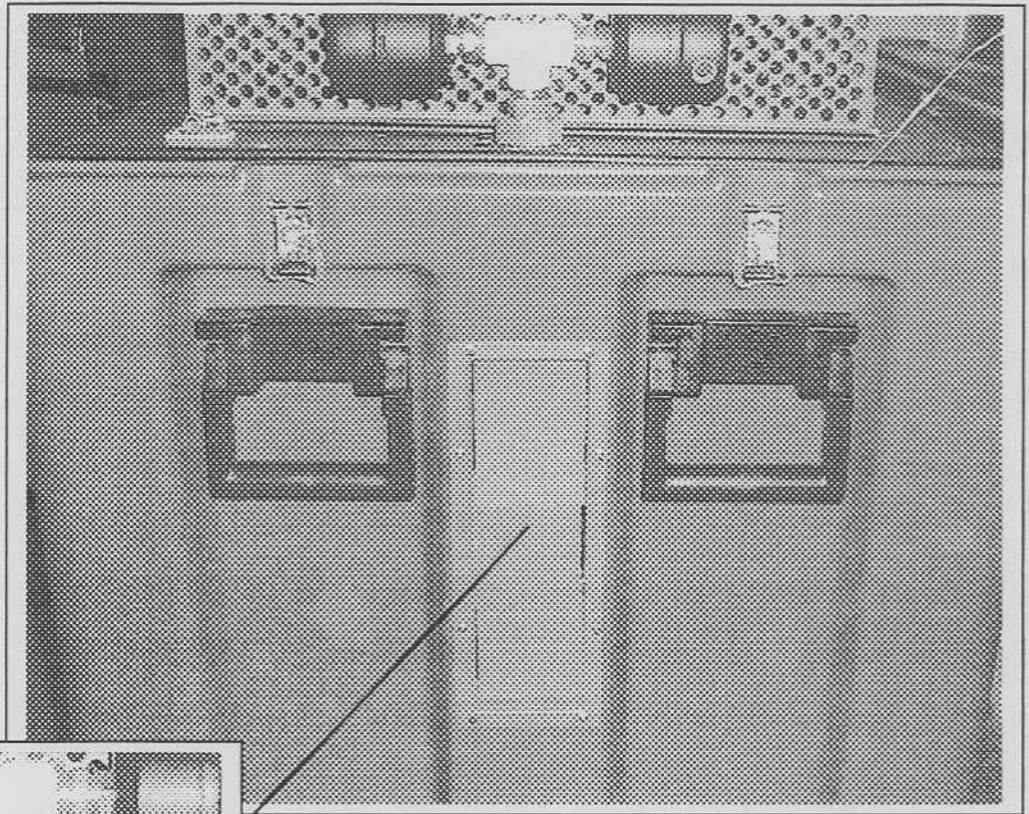
Photograph 32 POGS 3.3 Feed Compressor Outlet Filters Replacement
